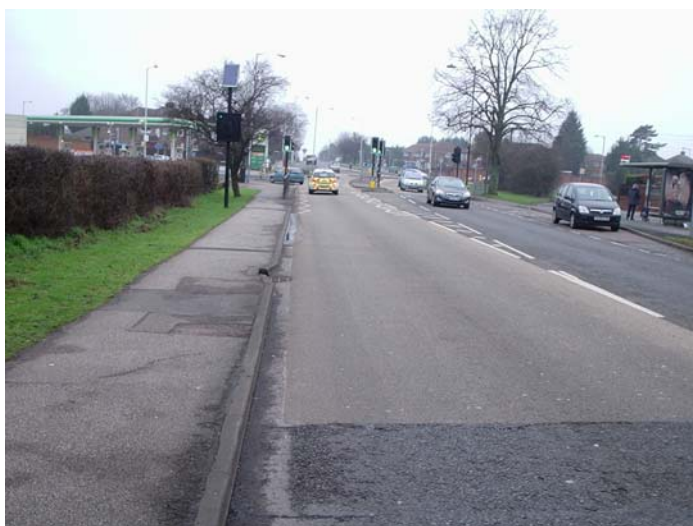
Skid resistant surfacing laid on the approach to a pedestrian crossing
